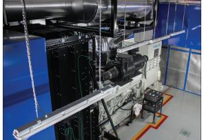
To mitigate sound a 30 to 35 dBa attenuation super critical NELSON silencer was used.
